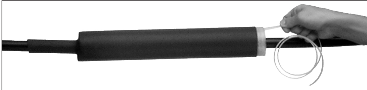
Removing the core
